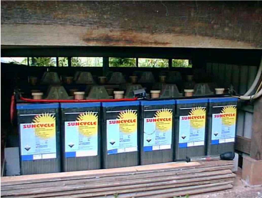
**Appendix 2 Fig 4** Battery located under a shed floor. Such locations (quite common in the Daintree) make routine maintenance and cleaning of the battery tops a very daunting task. At least the installer put the batteries in an appropriate plastic catch tray, which also stops organisms moving up and growing up between the battery cases, and the batteries are kept cool and well ventilated (by default). The de-sulphator is obvious on top of the batteries.
