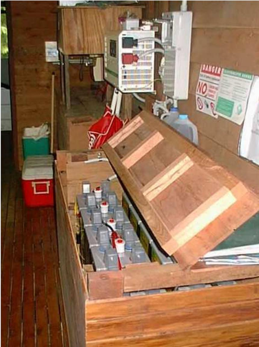
**Appendix 2 Fig 1** A basic system employing AS1100 batteries, a Trace Inverter, and a BPR4-NG controller. Not shown, Yanmar 5.5 KVA diesel generator, and 18 BP 75watt panels. This system was installed by the householder. The red and black wires running along the top of the batteries belongs to the desulphator. This system has been installed within the living space of the householder, and the batteries are separated from the remainder of the system in their own box.
