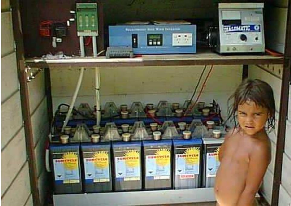
**Appendix 2 Fig 2.** A common style of installation, in this case employing AS 1100 flooded cells (24V) a fused DC disconnect, Selectronics SA31 inverter and a Woods Dialomatic battery charger, Prostar 30 regulator all installed in a lockable garden shed. Battery vents are directly below the top shelf. (not shown is a Lister 5KVA generator and 10 BP 75watt panels). The child is optional.
