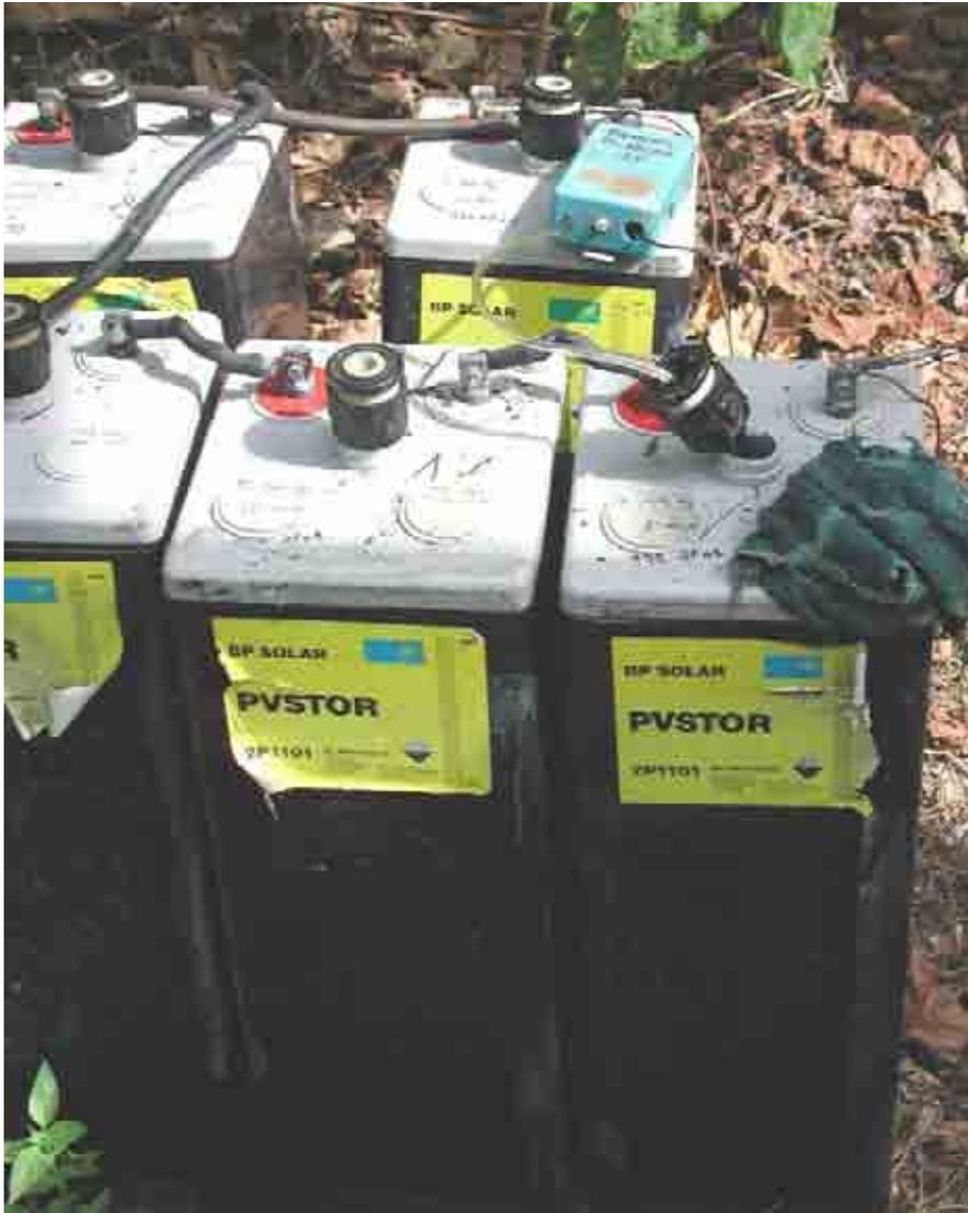
**Figure2** A battery driven bubbler (small blue box) with its output tube inserted into the side of a PVStor cell. These cells have been removed from the system, but are still useable, and are being trickle charged from the main Array while being held as spares for other failing systems in the area.
